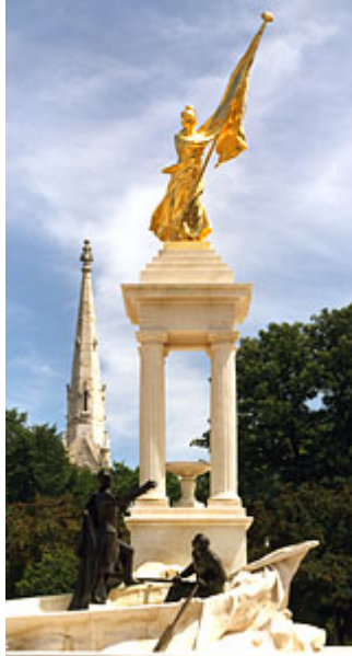
The Francis Scott Key Monument after conservation treatment. The monument received conservation treatment in the summer of 1999, when SAT Inc. cleaned the bronze and stone, replaced missing parts, and reapplied gold leaf. Photo: ©Ron Solomon.
